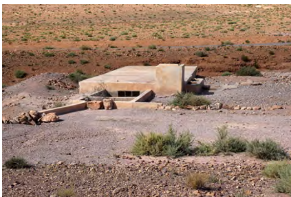
Fig. 72: Modern matfia (cistern) for the storage of rain water running off quickly. North of area AN1b, domain C, autumn 2015.
