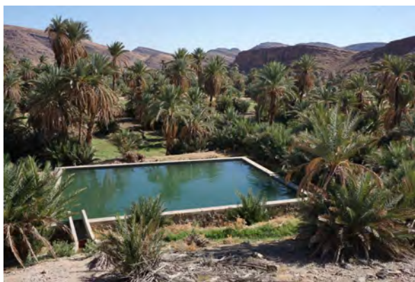
Fig. 157: Open cistern for irrigation of palm gardens near Aguerd on the lowermost Assif N'Innt. Domain C, area AS1i, autumn 2015.
