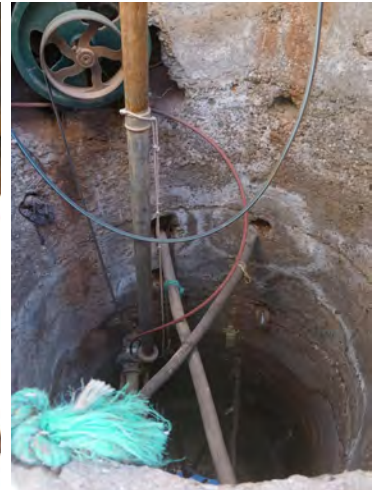
Fig. 92: Former draw well recently equipped with a motor pump. Wa-Ou-Nsamt, High Atlas Mountains, spring 2015.
