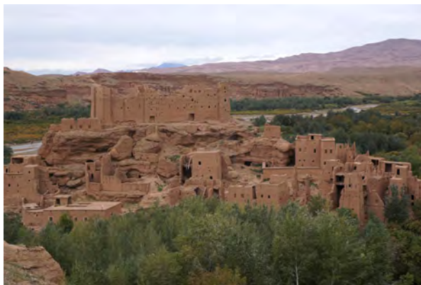
Fig. 193: Decaying Khsar north of El Kelâa des Mgouna, situated on a hill above Asif Mgoun. Foothills of the High Atlas Mts. in the background, view towards west. Area D2c, autumn 2015.
