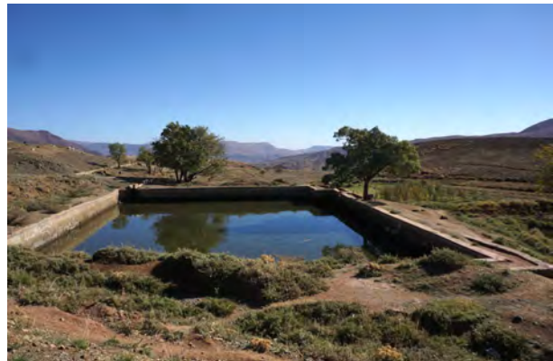
Fig. 222: Open cistern for the purpose of irrigation near village Tichkiouine. Area D5e, autumn 2015.
