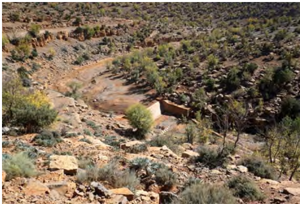
Fig. 415: Micro-dam that helps to branch irrigation channels from Oued Lakhdar. Near Tighremt 'Ighram N'Caid Ahansal', southwest of Ait M'Hamed, area O2, autumn 2015.
