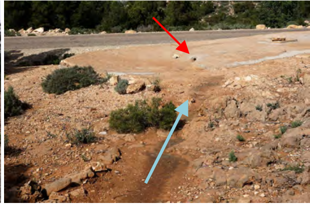
Fig. 442: Traditional matfia (cistern) from fig. 441, seen from the opposite side. The water flows in the direction of the blue arrow through the hole (red arrow) into the matfia. Jurassic carbonate plateau in the Atlantic Atlas Mountains, area WA1, autumn 2015.
