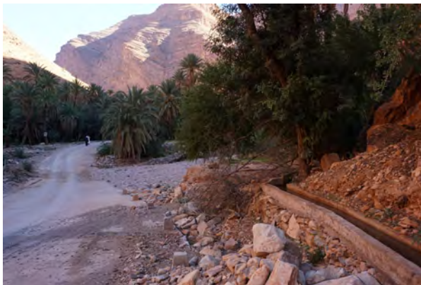
Fig. 139: Irrigation channel in the palm oasis near village Ighmir, fed by streams and sources in lateral valleys. Domain C, area AS1h, autumn 2015.
