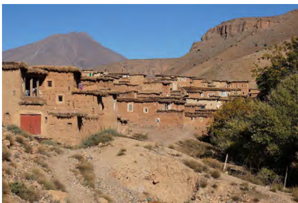
Fig. 124: Village Aït Ouanougdal, characteristic for the pisé-technique using stamped clay. Aït Bougoumez Valley, High Atlas Mountains, autumn 2015.
