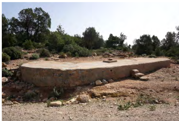
Fig. 101: Traditional matfia (cistern) for the storage of rain water running off quickly in the carstic underground on the carbonate plateau north of Imi Ouaddar. Westernmost High Atlas Mountains close to the Atlantic coast, autumn 2015.
