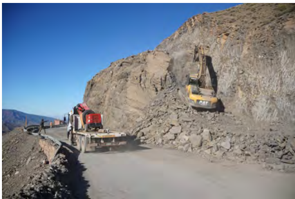
Fig. 91: Road construction site (broadening of the pass road). Area T1a, autumn 2015.
