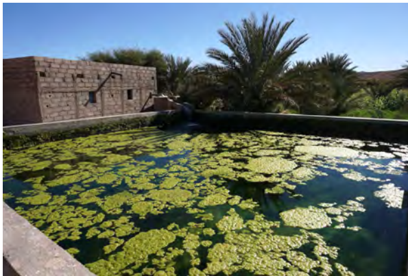
Fig. 210: Open cistern with a petrol driven groundwater pump for the irrigation of an isolated garden in the Akka Ighane – Tissint alluvial plain. Domain C, area AS4e, autumn 2015.
