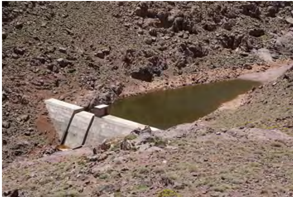
Fig. 43: Micro dam for irrigation and household water supply (see also fig. 42). Domain B, area JS3, spring 2015.
