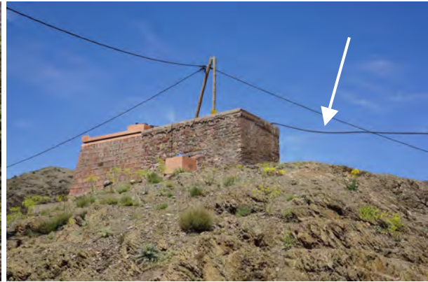
Fig. 137: Cistern filled with water by means of a plastic tube that is connected with a source (arrow). Tichka Valley, High Atlas Mountains, spring 2015.
