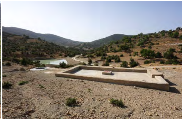
Fig. 444: Modern matfia (cistern) and small dam (background) on the Jurassic carbonate plateau in the Atlantic Atlas Mountains. Areas WA2a+b, autumn 2015.
