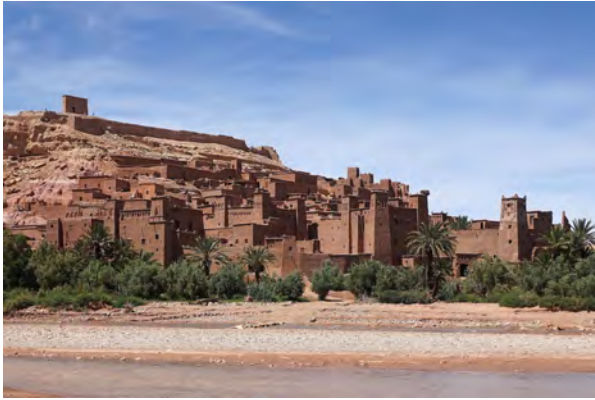
Fig. 130: Ksar Ait Ben Haddou in the lower Asif Ounila Valley is a United Nations World Heritage. It was built with the pisé-technique and is very prone to weathering. Despite of ongoing repair, its decay can hardly be stopped. Southern foothills of the High Atlas Mountains, spring 2015.
