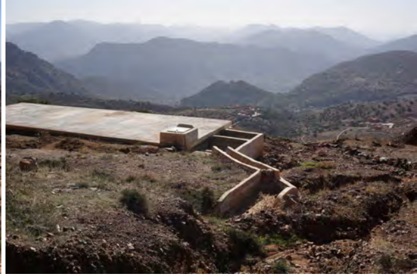
Fig. 33: Modern matfia (cistern) for the storage of rain water running off quickly. Near Tagezin, view towards southwest over Thmani and Tisi. Domain B, area Ma1c, autumn 2015.
