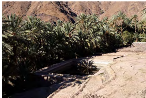
Fig. 187: Open cistern for irrigation in the Aguinane oasis. Domain B, area AS4a, autumn 2015.
