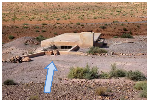
Fig. 102: Modern matfia (cistern) for the storage of rain water running off quickly on dry soils (direction of water flow see arrow). North of Souk El Had Azghar N'Irs, AntiAtlas Mountains, autumn 2015.
