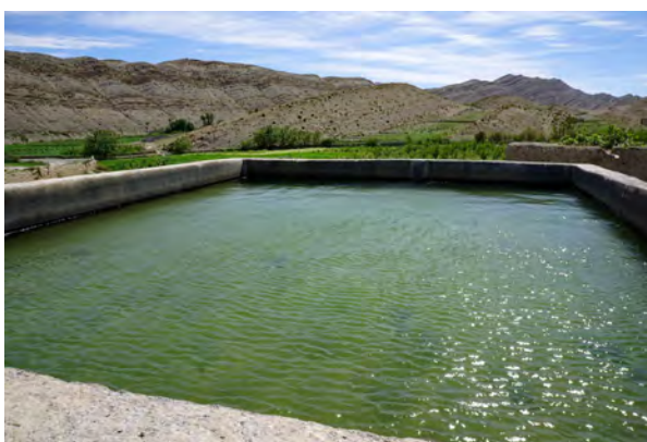
Fig. 289: Open cistern for the purpose of irrigation at Tamzazerte. Oued Taribante trough valley, area Z1c, spring 2015.
