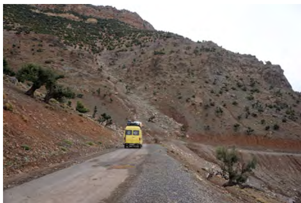
Figs. 104: Debris flow near Ait Hammodo due to deforestation of the slope. High Atlas Mountains, autumn 2015.
