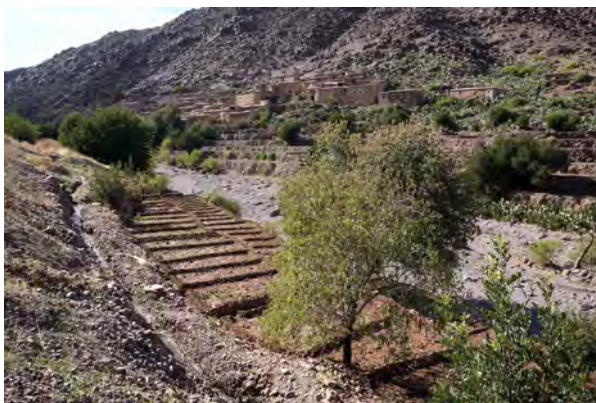
Fig. 84: Village Tingarf with a rare irrigation channel (left) and small, irrigated fields. Domain B, area AN1a, autumn 2015.
