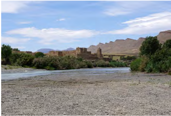
Fig. 298: Lower course of Oued Taribante in a broad trough valley, with the old Kasbah of Tamagourte. View up the valley, area Z1i, spring 2015.
