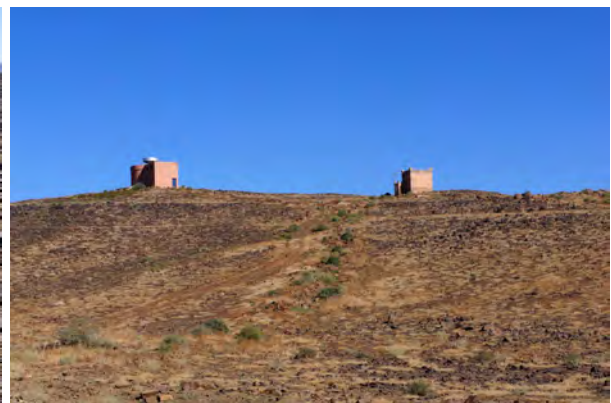
Fig. 15: A new (left) and an older (right) cistern for the water supply of villages on the foot of the mountains. Domain C, area JS1a, autumn 2015.
