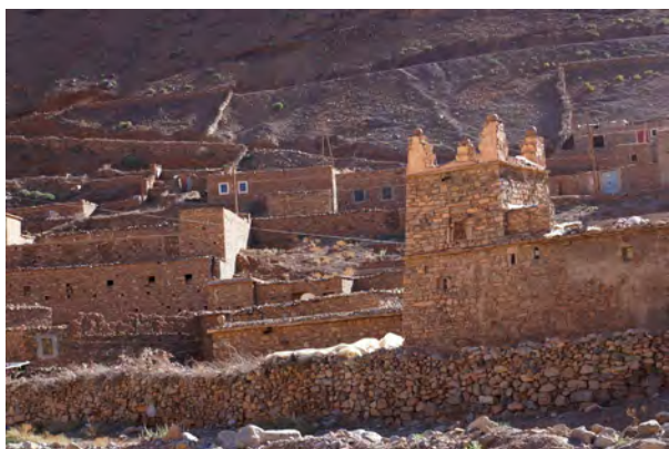
Fig. 123: Village Imi N'Tatellate (Ait Yacoub), one of the rare villages constructed fully with stone blocks that are not plastered. AntiAtlas Mountains, autumn 2015.
