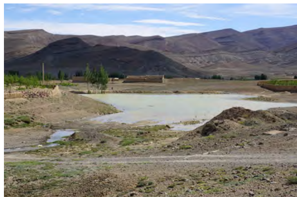
Fig. 100: Traditional micro dam for irrigation, made of mud, collecting water from small, episodic streams. Near Almgho, Assif Melloul Valley, High Atlas Mountains, spring 2015.
