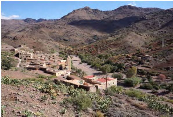
Fig. 82: Village Touadil with unusually many traditional houses in good condition. Ploughed, terraced fields for dry cultivation in the middle ground, view down the valley. Domain B, area AN1a, autumn 2015.
