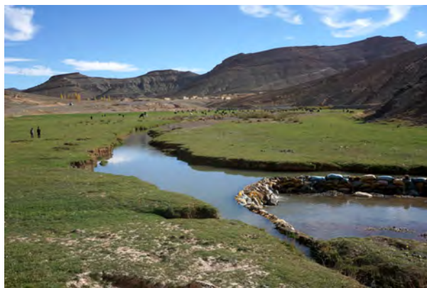
Fig. 80: Damming of Assif Melloul to supply irrigation channels on both sides near Tissila. High Atlas Mts., autumn 2015.
