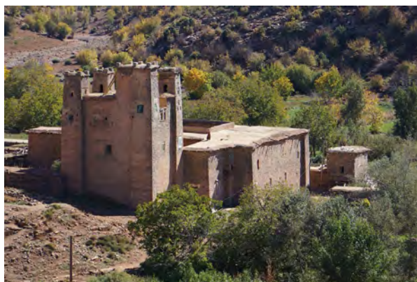
Fig. 126: Well-preserved and inhabited Tighremt 'Ighram N' Caid Ahansal' near Oued Lakhdar southwest of Aït M'Hamed, built with limestone blocks. High Atlas Mts., autumn 2015.
