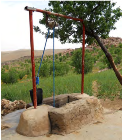
Fig. 90: Draw well for the irrigation of almond trees near Azoura. AntiAtlas Mountains, spring 2011.
