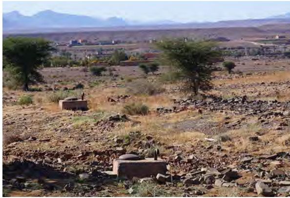
Fig. 16: Shafts belonging to a water pipe leading from the cisterns (fig. 15) down to the villages on the foot of the mountains. Domain D, area JS1d, autumn 2015.
