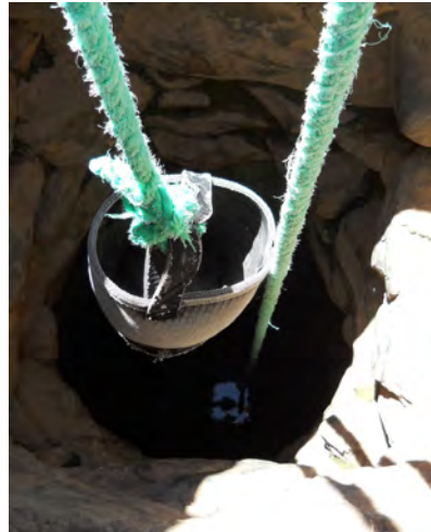
Fig. 91: Bucket in a draw well made of a truck tyre. AntiAtlas Mountains, spring 2011
