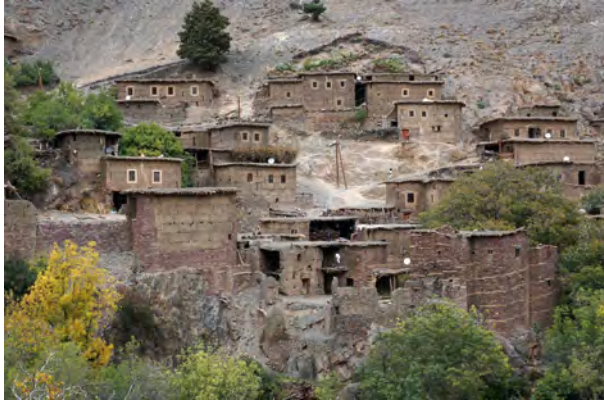
Fig. 125: Village Imizilen in the Megdaz Valley, where part of the houses are built with stone blocks and part with stamped clay. High Atlas Mountains, autumn 2015.
