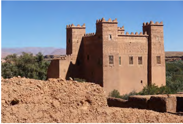
Fig. 128: Tighemt of Agafay, built with unburnt clay bricks and displaying ornaments in the upper part of the wall. Near Boumalne du Dadès, south of the High Atlas Mountains, spring 2015.
