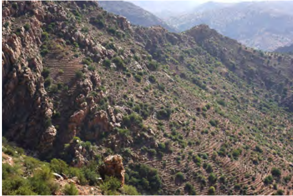
Fig. 16: Most of these artfully arranged terraces near Azouran and Tilian west of Tafraoute are about to disintegrate. Domain B, area Ma1c, autumn 2015
