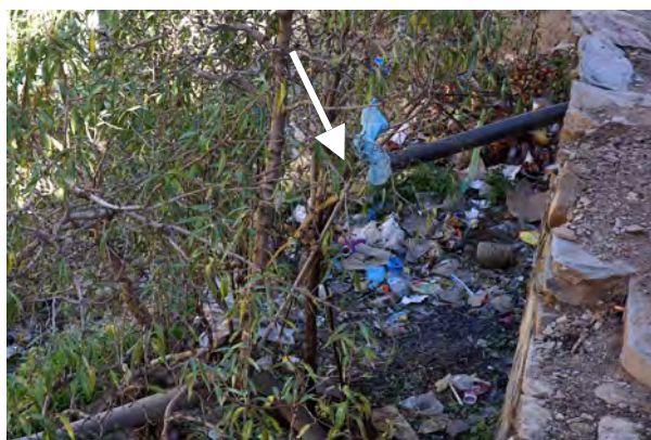
Fig. 142: Sewage pipe (arrow) and waste disposal in the village Aghbare in a lateral valley of Oued N'Fis Valley. High Atlas Mountains, autumn 2015.
