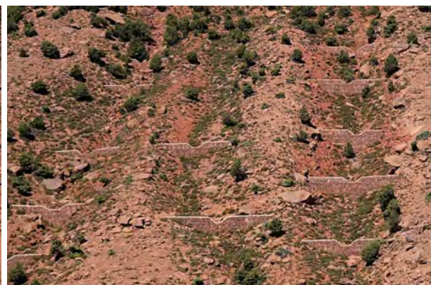
Fig. 430: Detail of fig. 429: Erosion gullies that developed in the deforested part of a steep slope are stabilized with micro-dams. East of Aït Ouiksane, area T2, autumn 2015.
