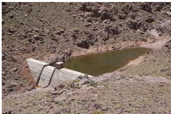
Fig. 99: Modern micro dam for irrigation and household water supply made of concrete, collecting water from rare rainstorms in a stream. North of Tizi N'Tazarine, Jebel Saghro, Spring 2015.
