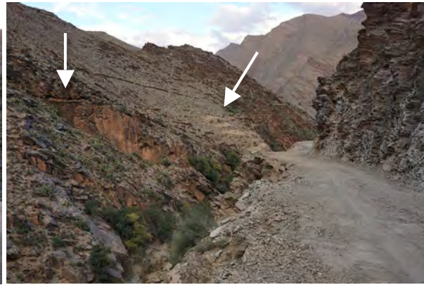
Fig. 139: Gorge of the Asif El Mehl with a new mud road. On the left hand side relics of terraced fields and of an old mule trail (arrows). View down the valley, area T5a, autumn 2015.
