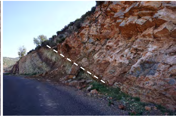
Fig. 448: Road cut showing the boundary between weak Triassic marls and overlying, harder Lower Jurassic limestones. Carbonate plateau in the Atlantic Atlas Mountains. Area WA2c, autumn 2015.
