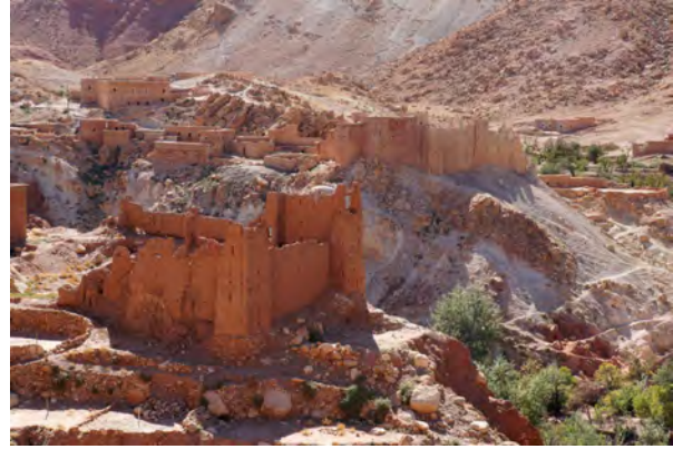
Fig. 129: Abandoned and disintegrated Tighemts of Tajenite that were built with the pisé-technique. Upper Asif Ounila Valley, southern foothills of the High Atlas Mountains, autumn 2015.
