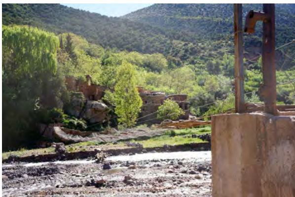
Fig. 110: Small village that is only accessible over a dilapidated suspension bridge during high water. Area T3b, spring 2015.
