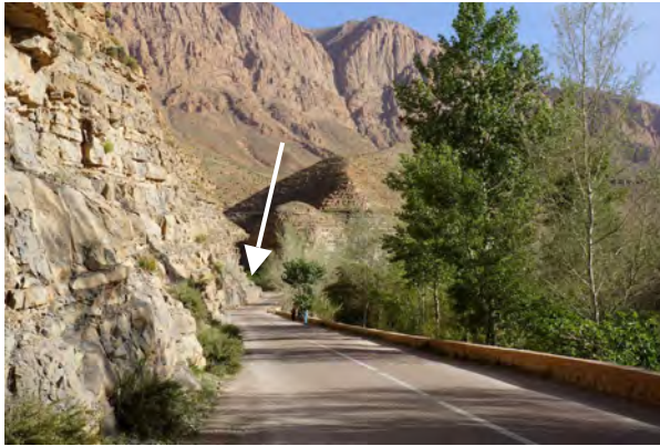
Fig. 386: Dadès valley near Tizguine in spring 2015. The arrow indicates the location of a heavy rockfall that occurred in summer 2015 (see fig. 387). View down the valley, area D1d.
