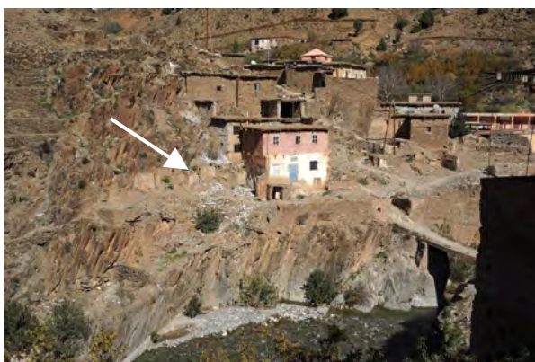
Fig. 118: Village Aghbare with a garbage heap (arrow); souk villages at the end of motorable roads are always situated "at the end of the modern world", suffering from its remnants that do not rot. Area T4a, autumn 2015.
