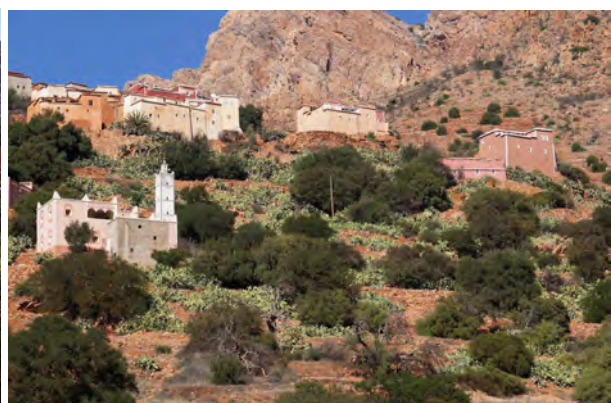
Fig. 31: Traditional houses in extraordinarily good condition in Azouran. Domain B, area Ma1c, autumn 2015.
