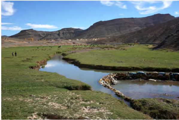
Fig. 314: Damming of Assif Melloul to supply irrigation channels on both sides near village Tissila. Asif Melloul trough valley, areas O3b, and O3d, autumn 2015.
