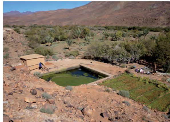
Open cistern and groundwater pump in the upper section of the Handour valley, Jebel Saghro.
