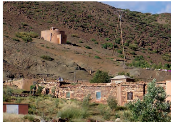
Cistern with a piping system in Argue, High Atlas.
