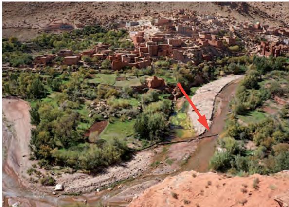
Asif Ounila with a small dam made of stones and sandbags to branch off an irrigation channel (arrow); Tiourassine, south flank of the High Atlas.
